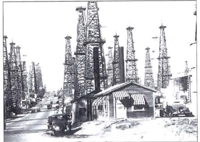
Figure 7b. Atlantic and 28th Street situated within the Signal Hill oil field circa 1930.
